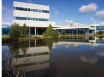
Danfoss Silicon Power, expansion cleanroom production building
