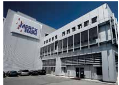
Merck Serono, expansion biotech production facility
