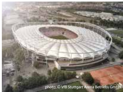
Mercedes-Benz Arena, TBM including operator responsibility
