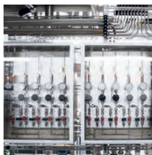
Ultra-pure media supply and disposal provided by ROM
